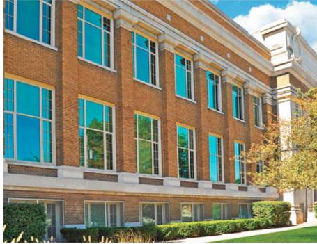
Projected and casement windows are hinged at the sides and swing outward. They are opened using levers or handles. EFCO offers a wide range of configurations that include project-in, project-out, casement and tilt-turn. EFCO's projected windows provide egress, ventilation, and window-washing functionality in addition to natural light.
