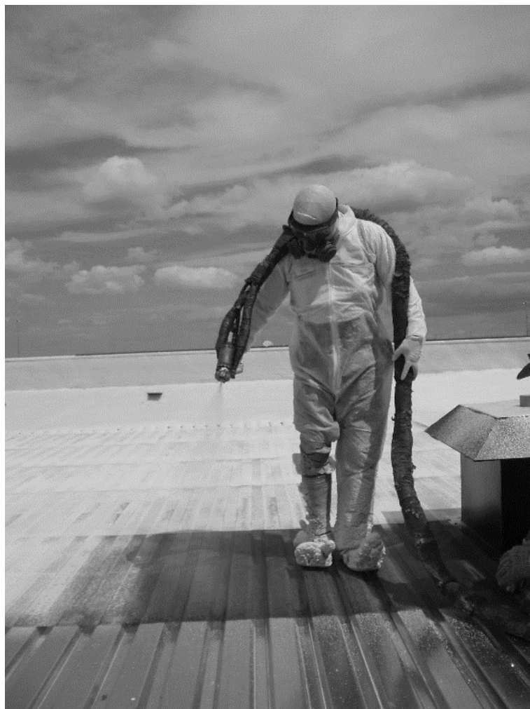
Spray Foam Roofing application.
