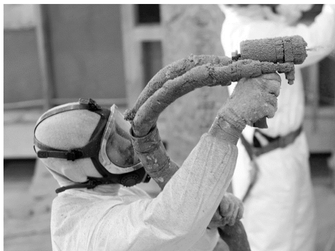
Spray Polyurethane Foam installation
