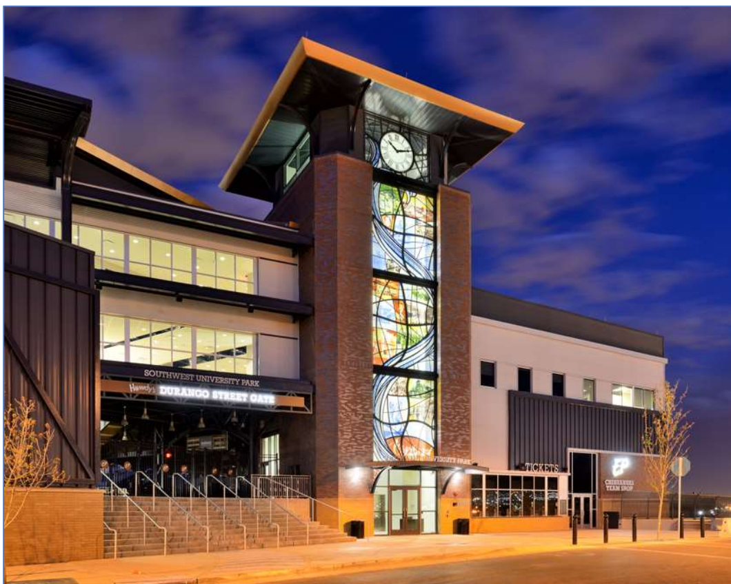
El Paso Clock Tower, Southwest University Park
