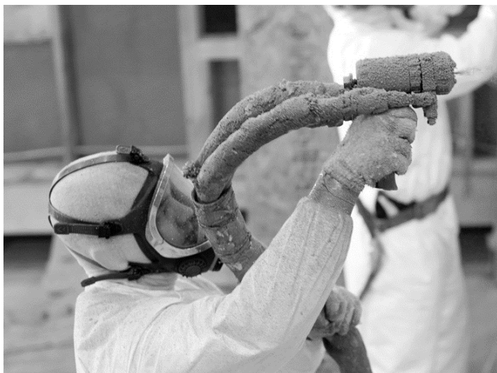
Spray Polyurethane Foam installation
