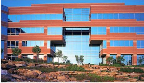
Used primarily for low to mid rise multi-family and mixed use buildings, window wall products provide the appearance of a traditional curtain wall system, but at a lower price point. Anchored at the head and sill at each floor and installed into the subframe, EFCO's window wall products can be installed from the building's interior.
