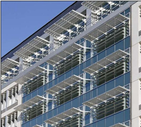
Typically assembled at the building site, a traditional stick-built curtain wall system is made up of a combination of horizontal/vertical mullions, glass, and is capable of multi-floor spans. Available in a variety of depths, profiles, and finishes, Wausau's relatively lightweight, weathertight traditional curtain wall systems provide a cutting-edge combination of design and performance, including thermal, hurricane and blast resistance.
