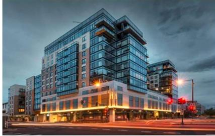
The unitized curtain wall is fabricated, assembled, and glazed inside the factory, allowing the erector to reduce their labor by focusing on installing already built units. Unitized curtain wall systems are fast becoming the preferred method for enclosing a building. EFCO’s unitized curtain walls can meet a range of applications found throughout the U.S.
