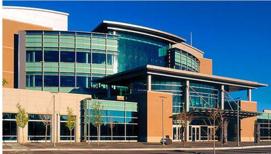
Typically assembled at the building site, a traditional stick-built curtain wall system is made up of a combination of horizontal/vertical mullions, glass, and is capable of multi-floor spans. Available in a variety of depths, profiles, and finishes, EFCO's relatively lightweight, weathertight traditional curtain wall systems provide a cutting-edge combination of design and performance, including thermal, hurricane and blast resistance.
