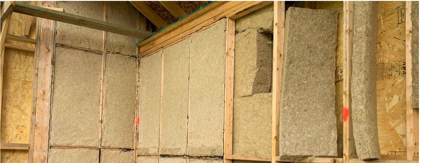
Photo 1. Installed Profib™ Mat insulation panel
