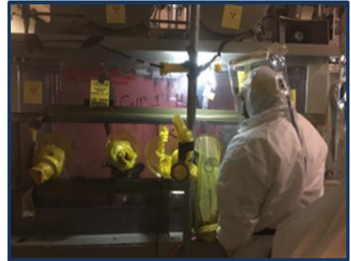
Application of Fire Resilient Fixative in 235-F PUFF Facility
