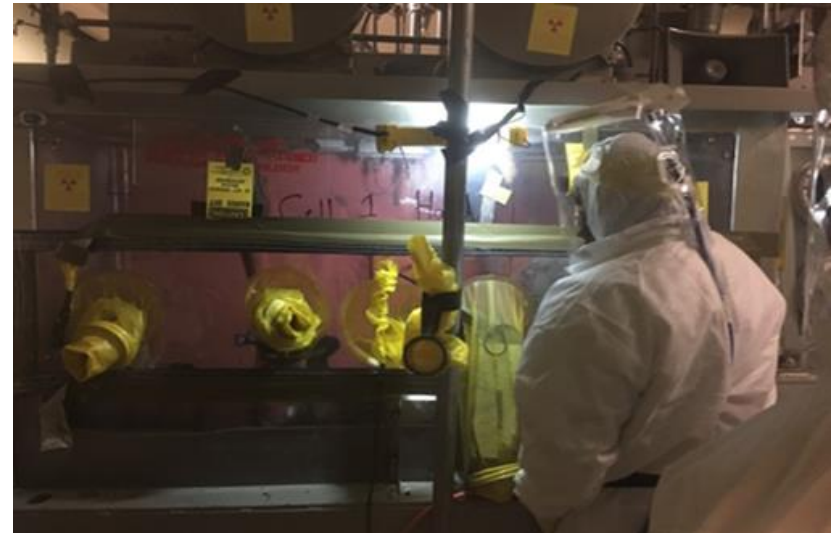
Application of Fire Resilient Fixative in 235-F PUFF Facility
