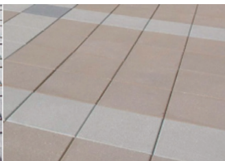
Segmental concrete paving slabs
